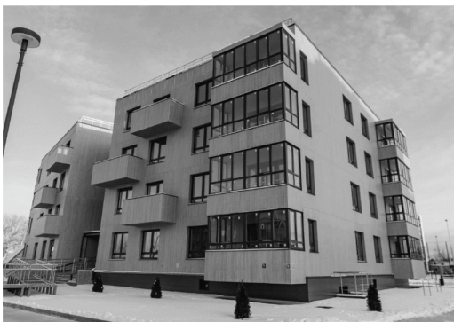
Fig. 1. Multi-storey residential buildings made of CLT panels in Russia
