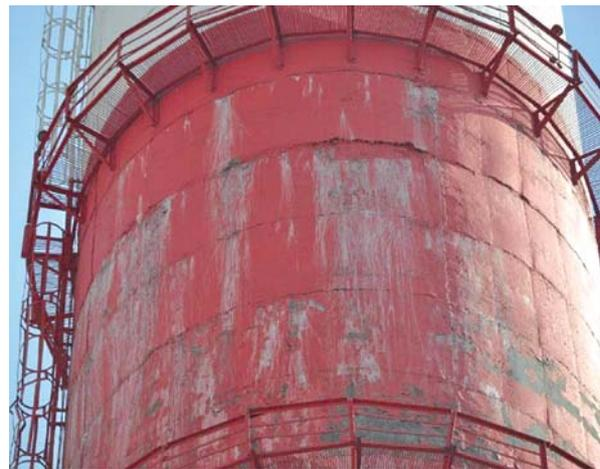
Fig. 4. Leaching process of free lime through weakened concrete sections
