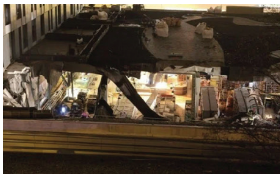
Fig. 4. Collapse of the shopping centre “Maxima”, Riga, 21.11.2013 7
