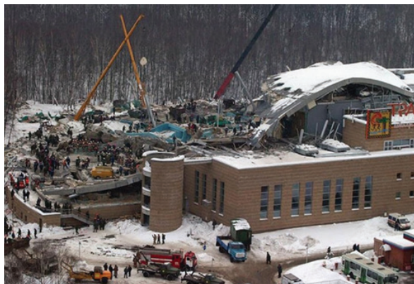
Fig. 1. Collapse of the building of the water park “Transvaal-park”, Moscow, 14.02.2004 1
