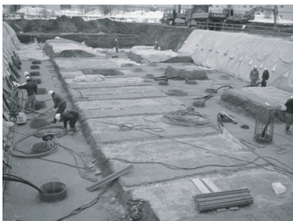
Fig. 3. Layout of installed 51 steel foundation piles and inserting of two sets of U-tubes, Sapporo city university, Japan [7]
