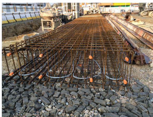
Fig. 1. Photo of the pipe cages used in the slurry walls at Cleunay station in Renne, France [3]
