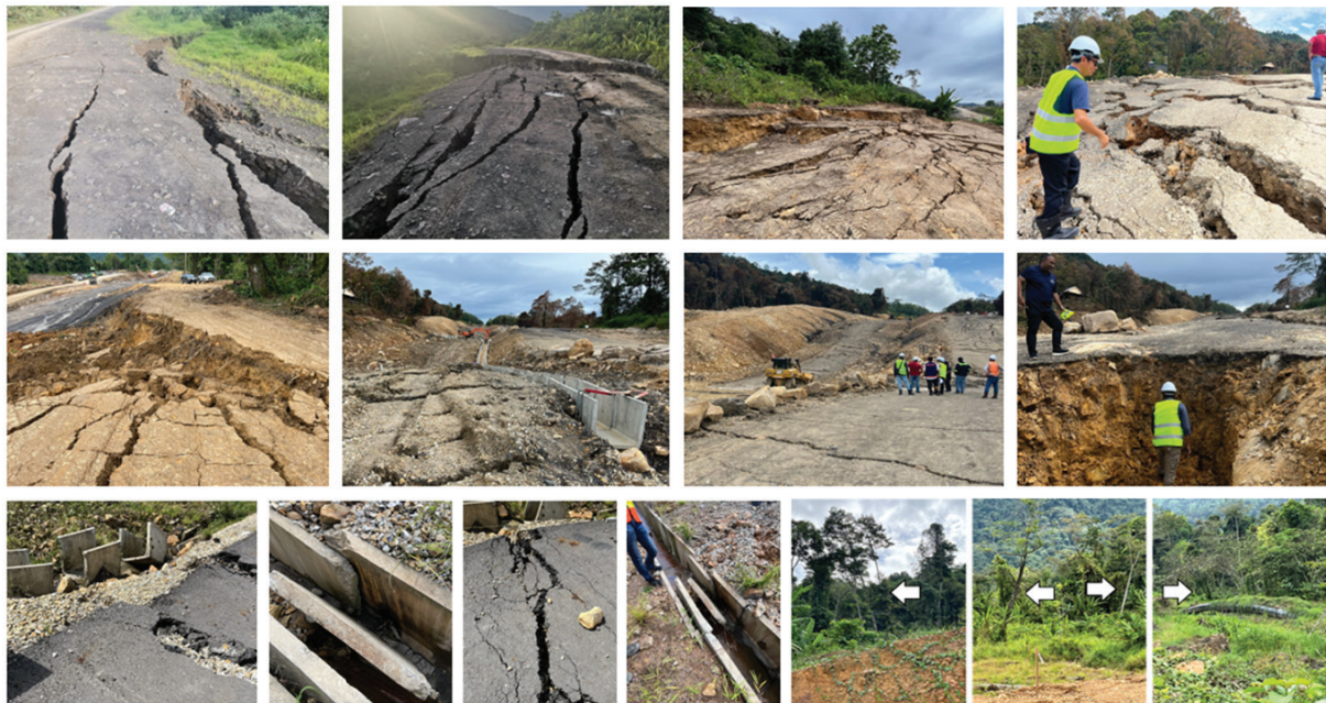
Fig. 5. Movement of ground during construction on site
