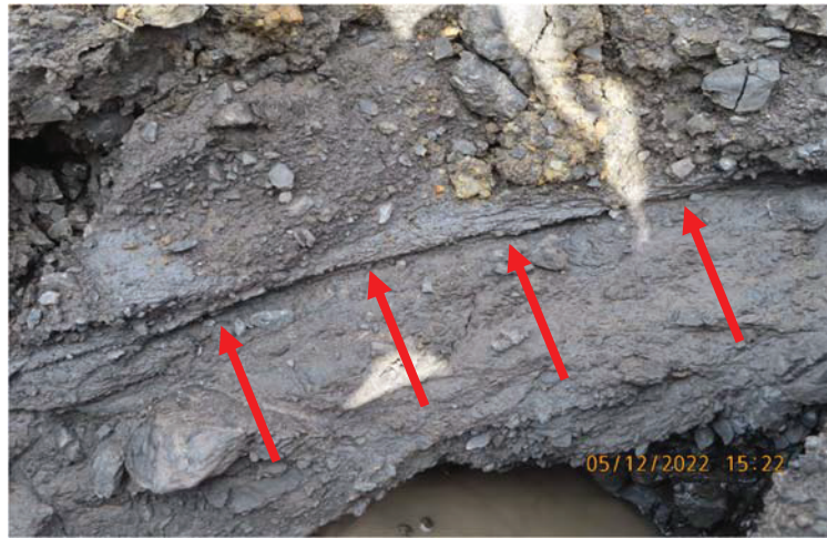
Fig. 6. Deposition of Mud seam layer form at the intersection of two different permeability layers
