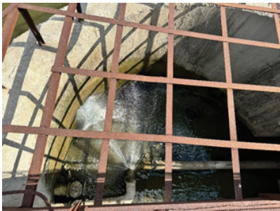
Fig. 7. Breakthrough of the mine spillway pipe at the Mikhailovsky I reservoir
