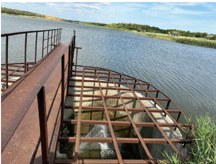
Fig. 8. Upper slope of the dam, shaft spillway
