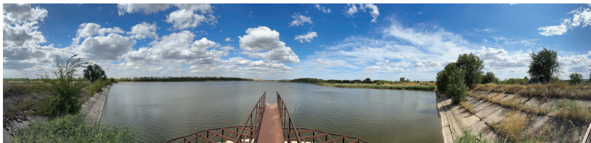
Fig. 1. View from the upper slope of the dam, shaft spillway of the Mikhailovsky I reservoir
