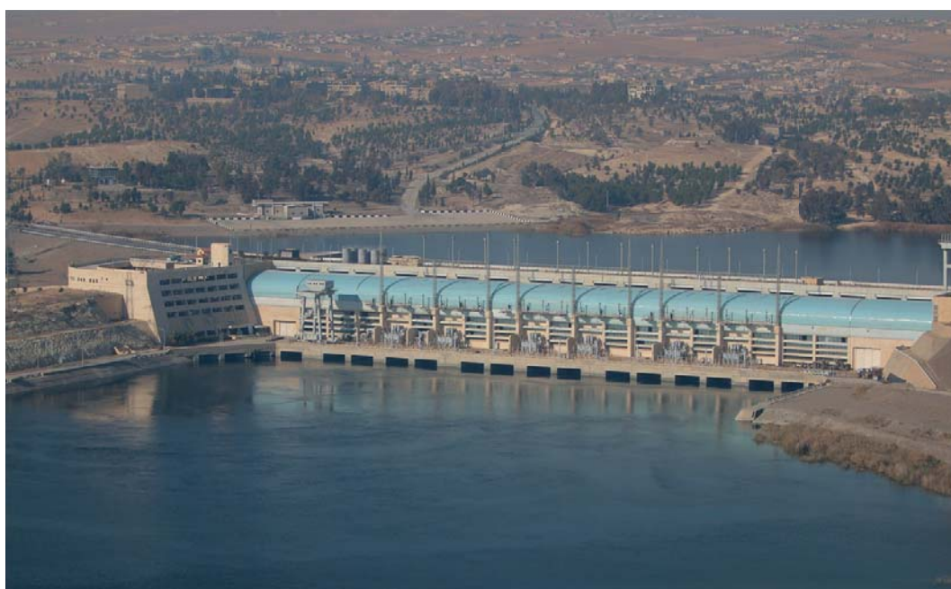
Fig. 1. The riverbed structure of the Tishrin HPP
