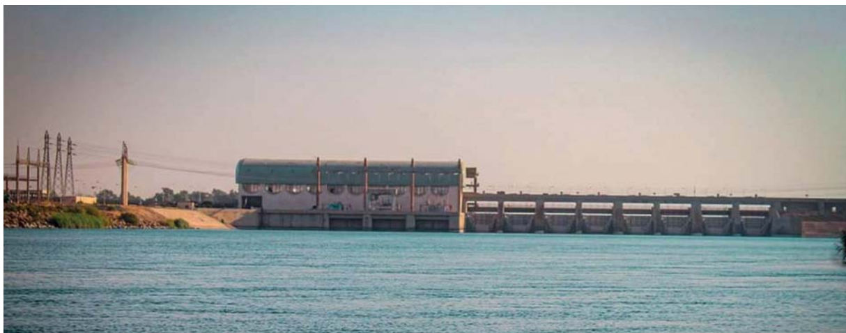
Fig. 3. View of the riverbed pressure structure at the Al-Baas HPP
