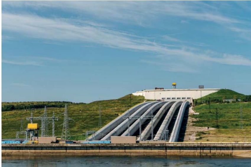
Fig. 4. View of the PSPP head building from the downstream side
