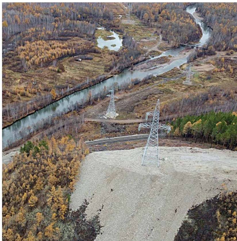
Fig. 1. The descent of the 220 kV single-circuit overhead line “Mogoch – Zilovo” from the hill and its crossing of the Trans-Siberian Railway and the freezing Amazar River (Transbaikal region, September 2022)
