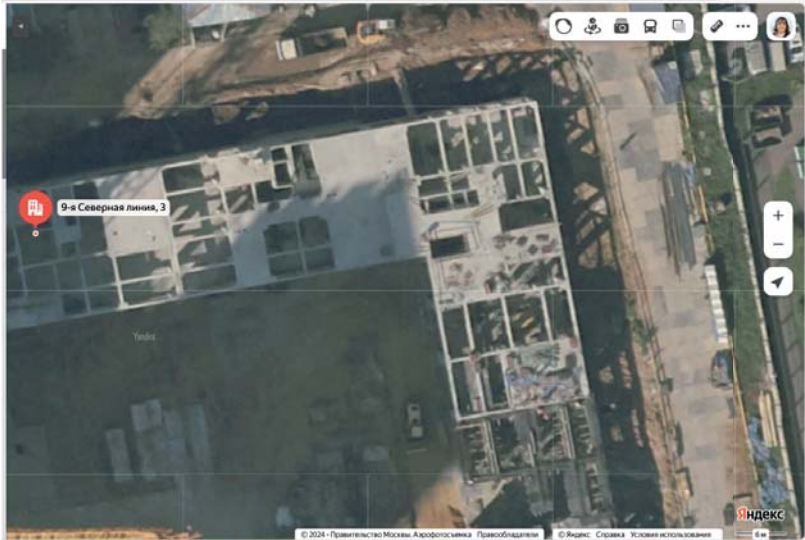
Fig. 7. Construction of storeys
