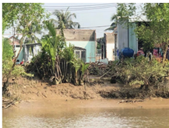
Fig. 1. Washout on the bank of the Saigon River
