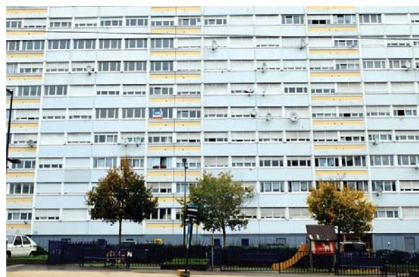
Fig. 3. An example of the renovation of a high-rise building in France under the National Urban Renewal Programme
