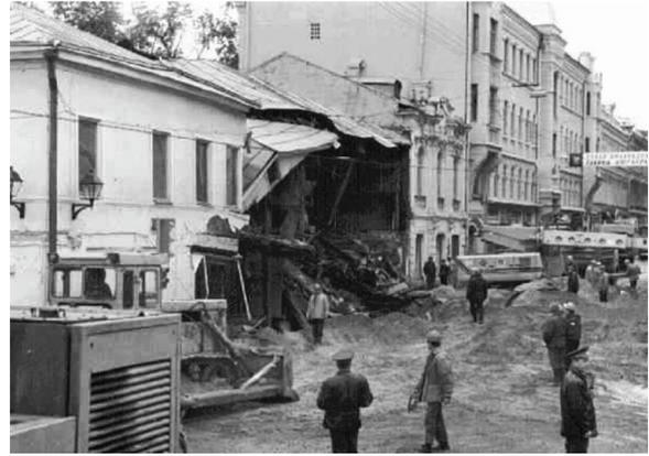
**Fig. 1.** A building and a street carriageway destroyed by a suffosion collapse sink formed as a result of hydraulic failure of water-saturated sands and their removal into a tunnel under construction (Moscow, 1998). Photo by V.P. Khomenko
