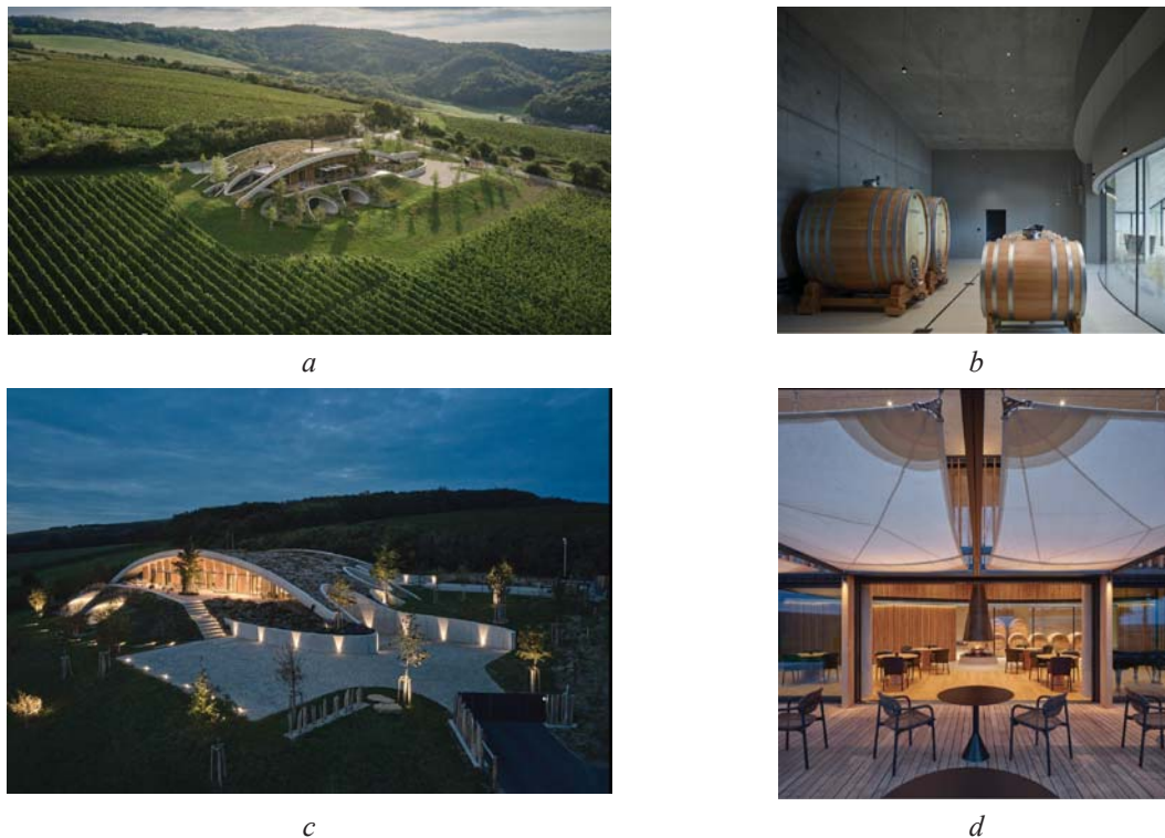
Fig. 6. Architectural solutions of Gurdau winery, Czech Republic (architect Ales Fiala): a — bird’s eye view; b — Interior of wine storage; c — exterior in the evening; d — interior of public area 5
