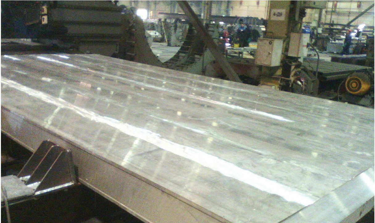
Fig. 9. Friction stir welding of an orthotropic slab on the bench
