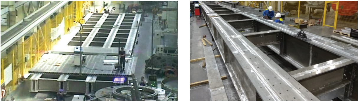
Fig. 16. Control assembly of span elements at the factory
