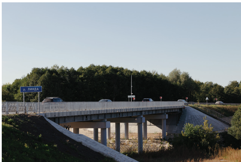
Fig. 21. Traffic on the aluminium alloy road bridge over the Linda River
