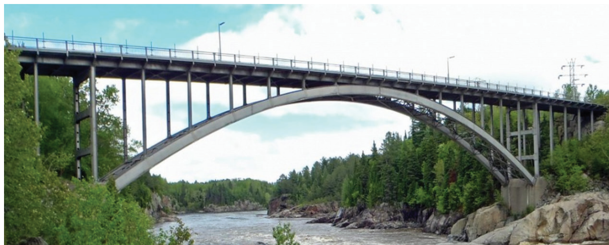
Fig. 1. Arvida Bridge, Canadian province of Quebec, centre span 88.4 m
