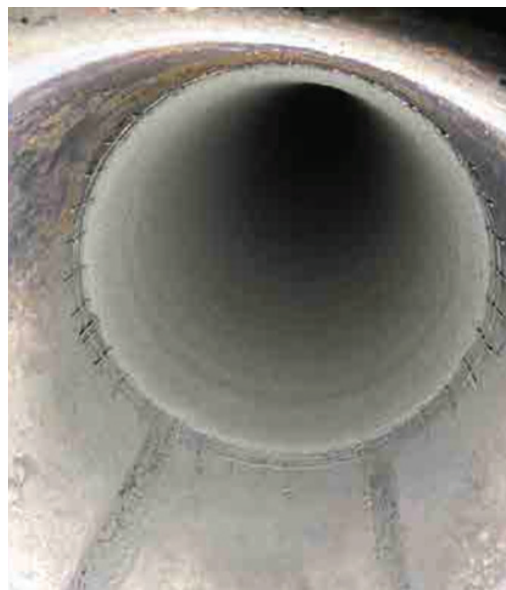
Fig. 2. Fragment of the “Arm-Pipe” protective coating applied to the purlins
