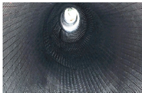
Fig. 3. Internal reinforcement of the pipeline with a mesh (grid) made of composite materials
