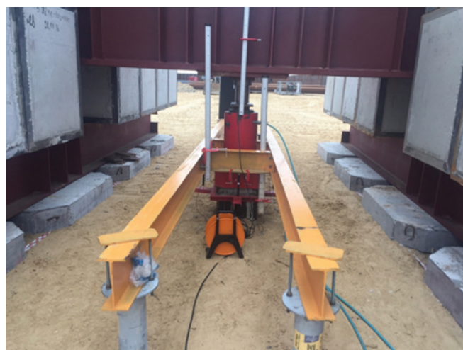
Fig. 3. Equipment for loading precast concrete joint piles
