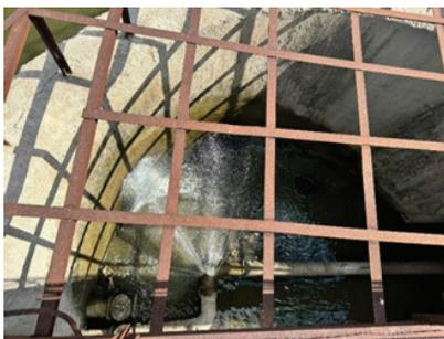
**Fig. 7.** Breakthrough of the mine spillway pipe at the Mikhailovsky I reservoir
