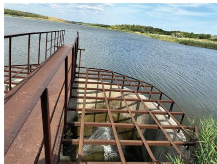
**Fig. 8.** Upper slope of the dam, shaft spillway
