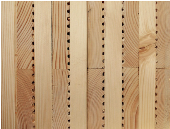
Fig. 3. The cross section of an MHM panel
