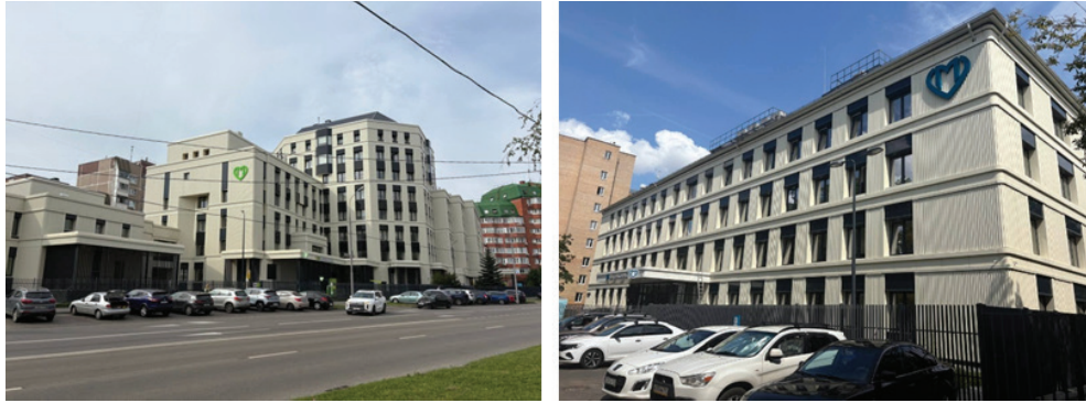
Fig. 6. Moscow polyclinic buildings renovated to a uniform standard
