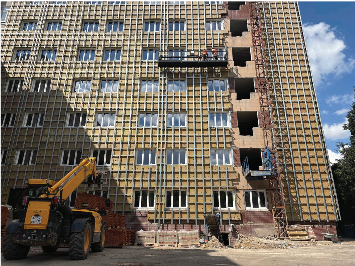
Fig. 3. Fragment of the facade of the facility where work is being carried out to install a curtain wall system
