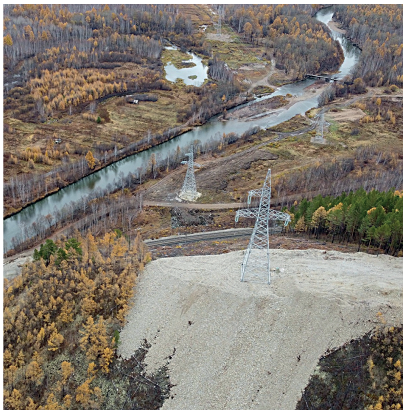
Fig. 1. The descent of the 220 kV single-circuit overhead line “Mogoch – Zilovo” from the hill and its crossing of the Trans-Siberian Railway and the freezing Amazar River (Transbaikal region, September 2022)
