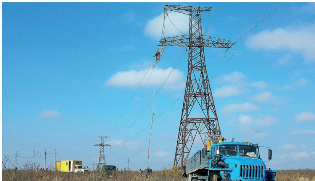
Fig. 3. Reconstruction of the 220 kV “Afipskaya – Krymskaya” overhead line, involving the replacement of old ASO-300 conductors with high-temperature GTACSR 217/49 conductors manufactured by the Japanese company J-Power Systems, using modern “tension-assisted installation” technology [12]
