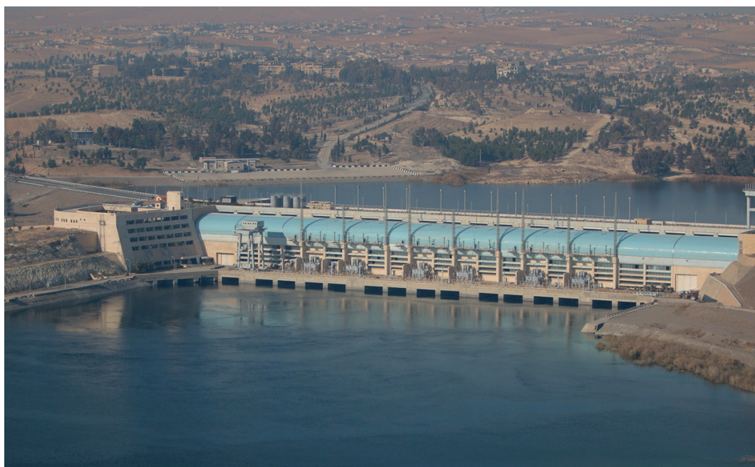
Fig. 1. The riverbed structure of the Tishrin HPP
