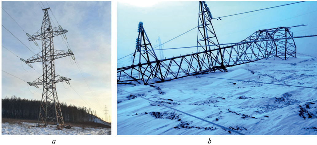
Fig. 2. Examples of damage and failures in power line structures: a — pre-failure tilt of an U220-1 anchor-corner support caused by frost heave of the foundations due to unanticipated freezing of the subsoil (Transbaikal region, December 2022); b — one of two fallen intermediate single-chain supports of type 2P220-1-6.8 due to wind loads exceeding design values (Irkutsk Region, Nov 2019)
