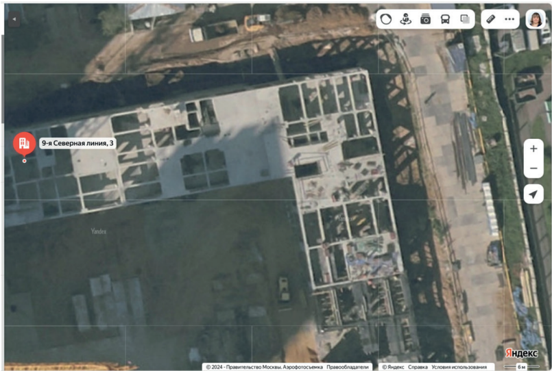
Fig. 7. Construction of storeys
